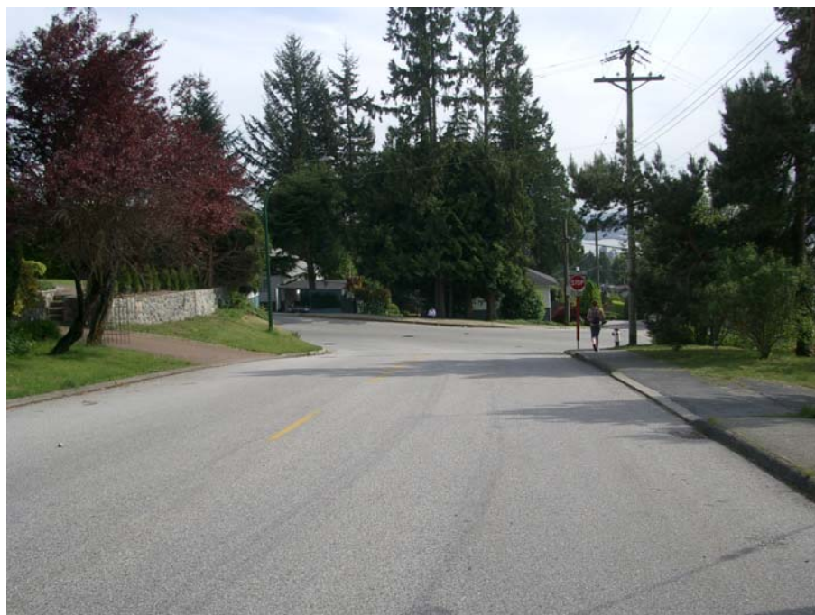
FIGURE 2.2 SMOOTH PAVEMENT ON NORTH LEG
