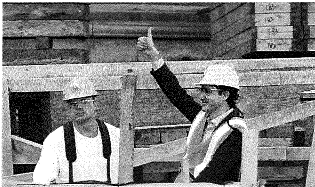
Justin Trudeau gestures to workers Tuesday as he tours the West Block construction site on Parliament Hill. Trudeau will become Canada's new prime minister at a swearing-in ceremony today. ADRIAN WYLD, THE CANADIAN PRESS
