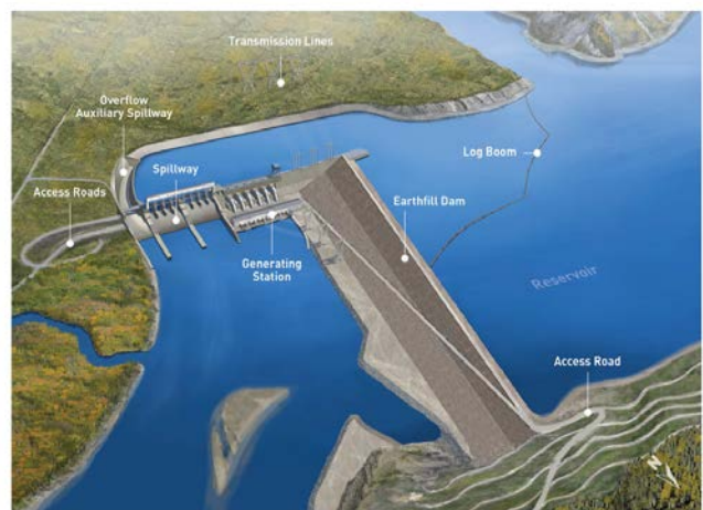
Picture X 2 Upgraded Dam (Christy Clark)
