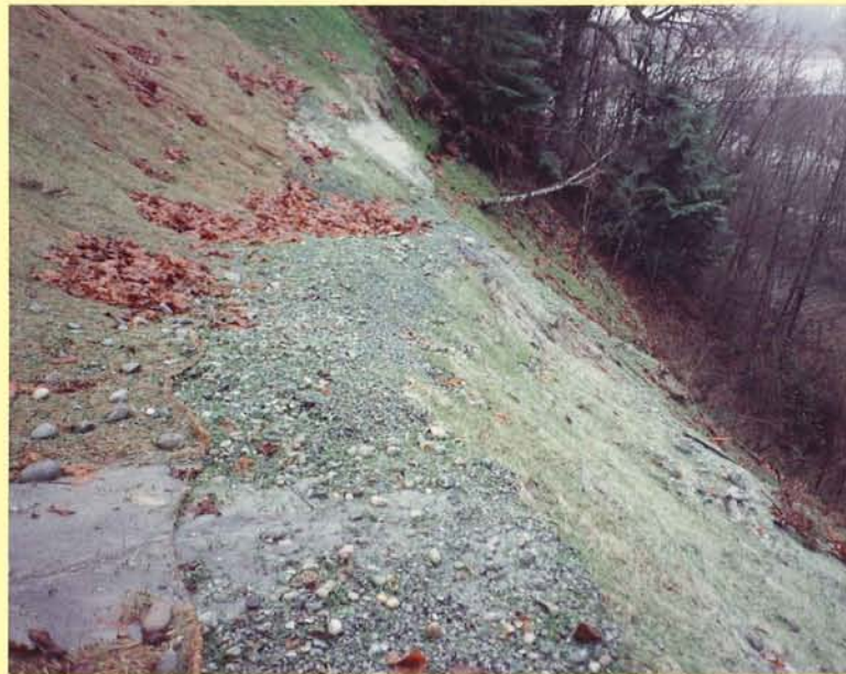
Photo 15 - Bench at toe of flattened slope above powerhouse.
