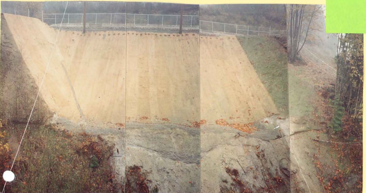
Photo 14 - As above on completion of stabilization
