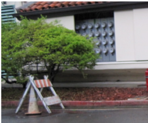
Smart meters newly installed Image source: OTLB (2011).
