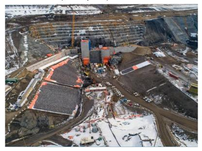
Figure A-6 Arial View of the Diversion Tunnel Outlet Portals and the Temporary Fish Passage Facility under Construction (February 2020)
