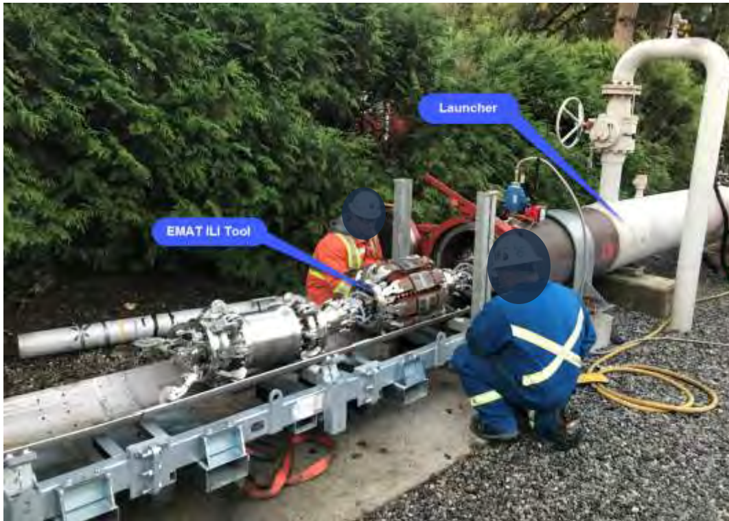
1 Figure 4-2: EMAT ILI Tool being Inserted into a Launcher
