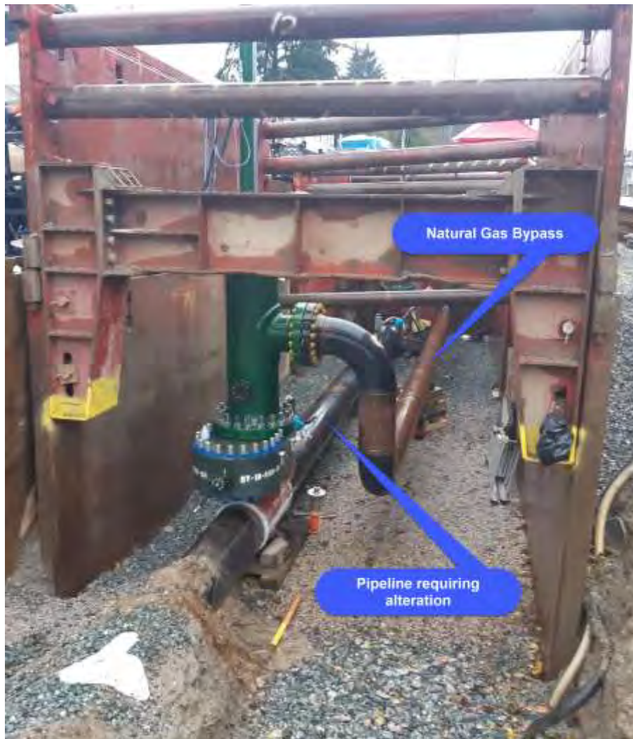
1 Figure 4-1(a): Example of a Pipeline Alteration with Natural Gas Bypass – Before Cut Out
