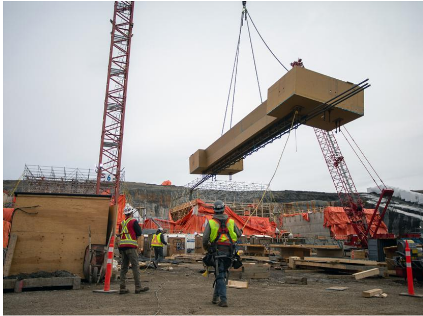
Figure A-1 Crews use a crane to lift formwork for placement at the spillway headworks (April 2021)
