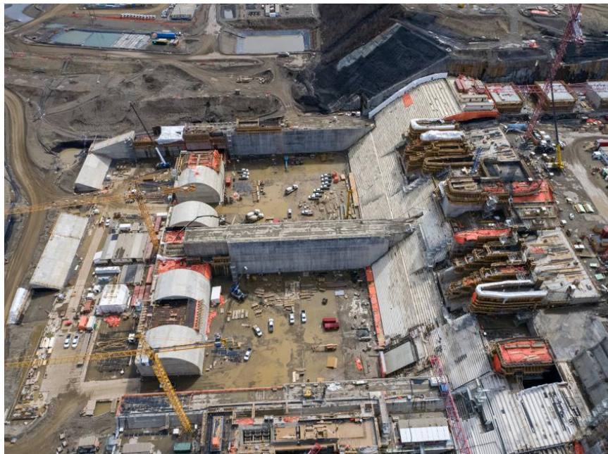
Figure A-2 The spillways, headworks and stilling basins (April 2021)
