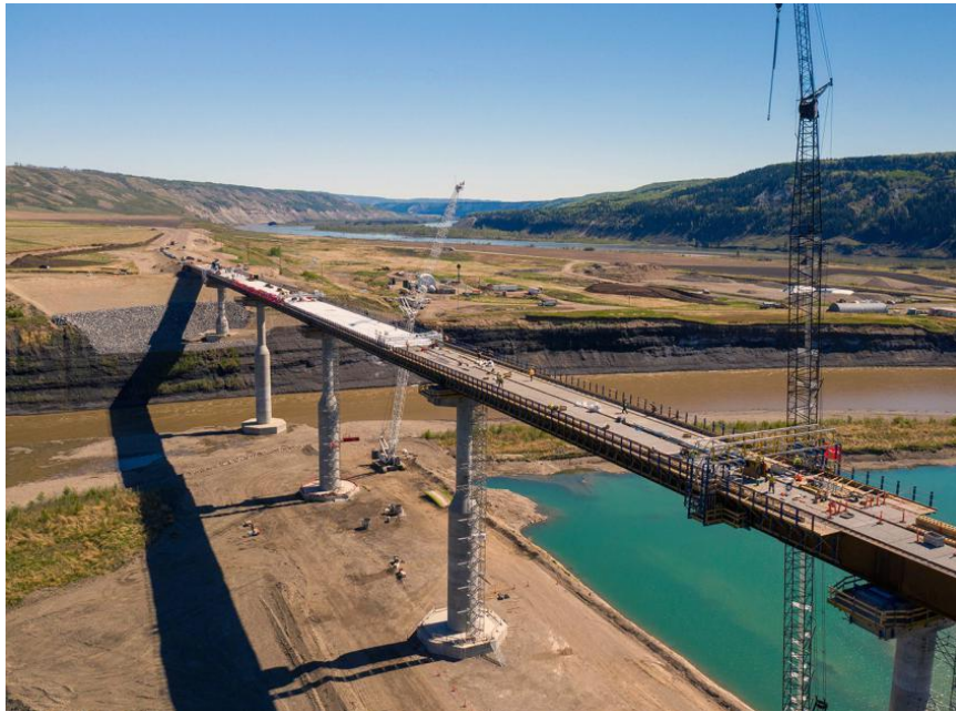
Figure A-6 Halfway River bridge showing cast-in-place bridge deck construction. The new bridge is over one kilometre long (May 2021)
