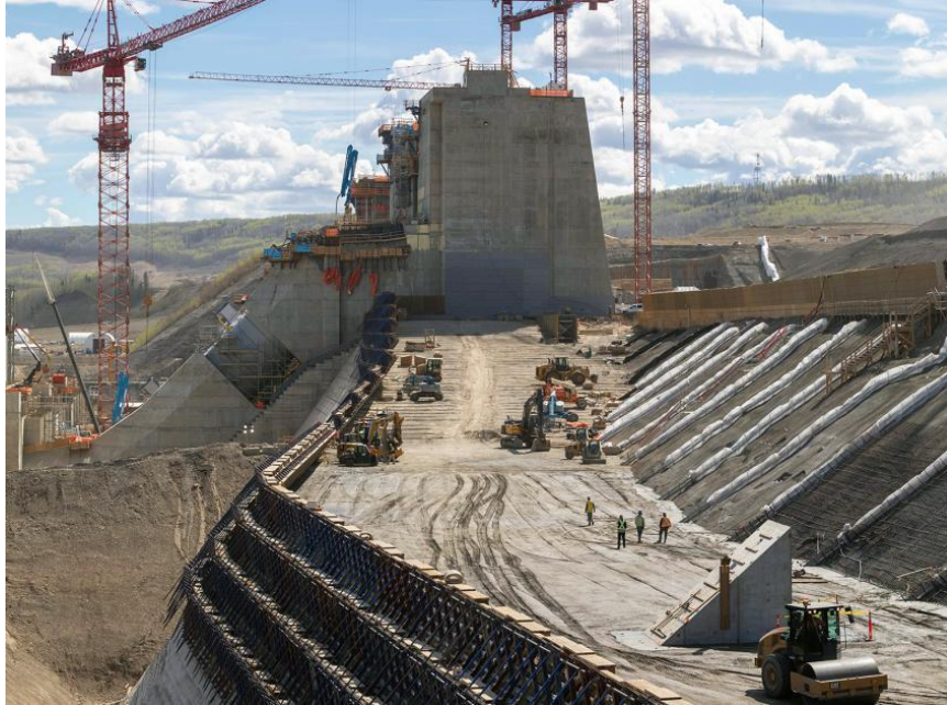
Figure A-5 Crews place roller-compacted concrete on the dam and core buttress (May 2021)
