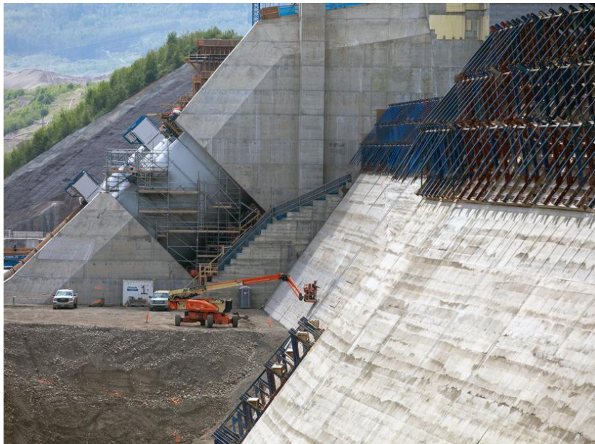
Figure A-10 Workers inspect the roller-compacted concrete at the dam and core buttress after the formwork is removed (June 2021)
